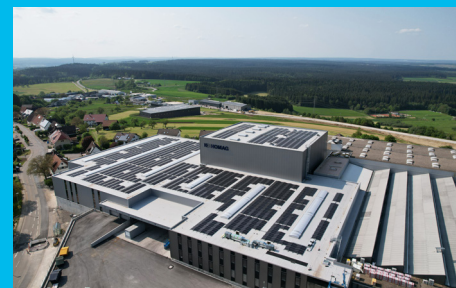
Photovoltaic system in Schopfloch
